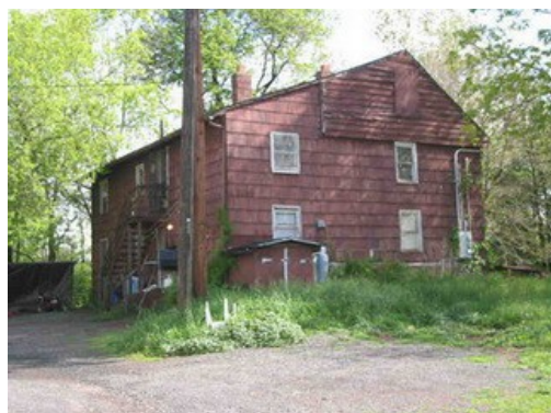
Recently torn down on the turnpike behind Blue Lobster
